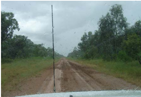
Light gravel over sandy base after rain and one light vehicle
