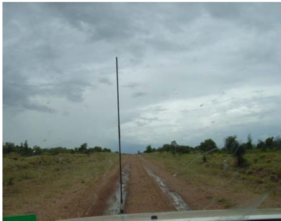
Light gravel over sandy base after rain and one light vehicle
